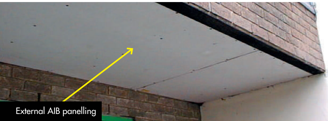
AIB soffit board
