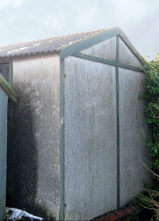
Asbestos cement panels and roof sheets
