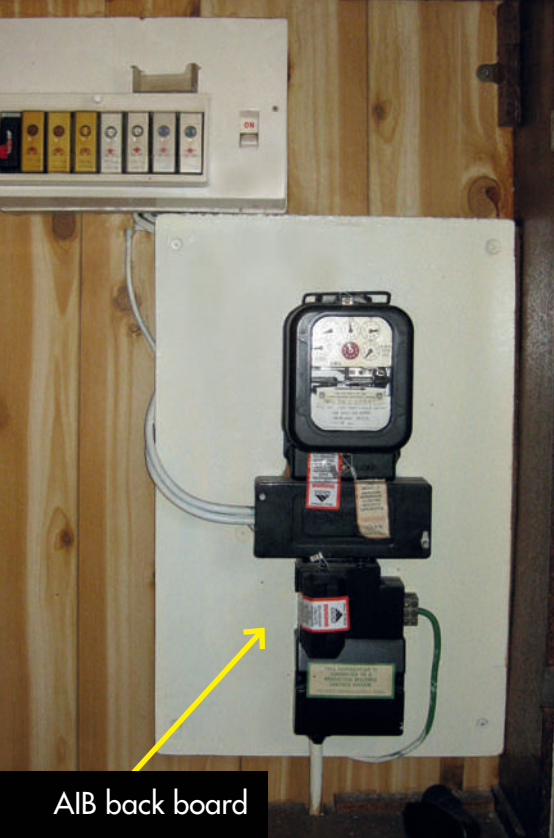
Asbestos flash guard
